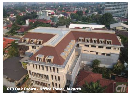
CT3 Oak Brown - Office Tower, Jakarta
